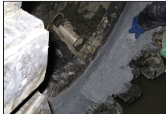
Applying ARC BX1*
